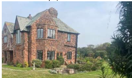
Blundellsands Hall similar featured bay and chimneys (more viewable from coast)
